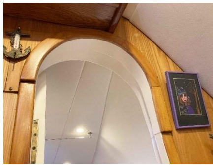
Reinforced cut out structural bulkhead starboard side
